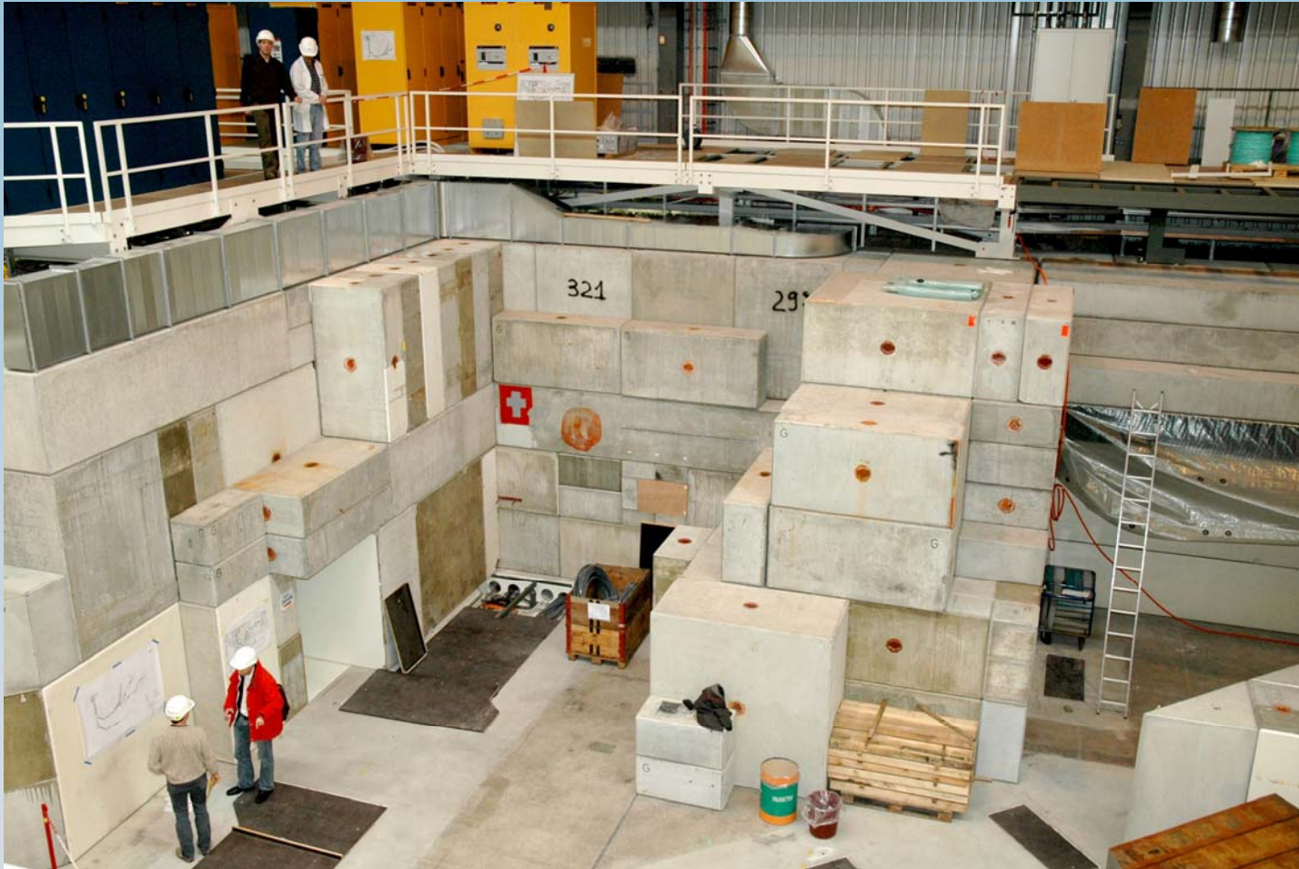
PROSCAN Site at Banding Magnet (Test Area)
