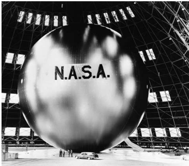
Static Inflation Test of 135 Ft Satellite In Weeksville, NC NASA Langley Research Center 6/28/1961 Image # EL-1996-00052
