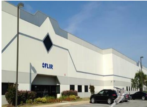
Elkridge, MD, US: Ground Vehicles
